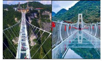
The bridge will have a 5-metre-wide steel deck for two-wheelers and 1.5-metre-wide glass walkways on both sides for pedestrians. The
