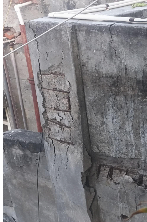
Image 11 : Showing Severe Damage to the column due to this reinforcement got corroded.
