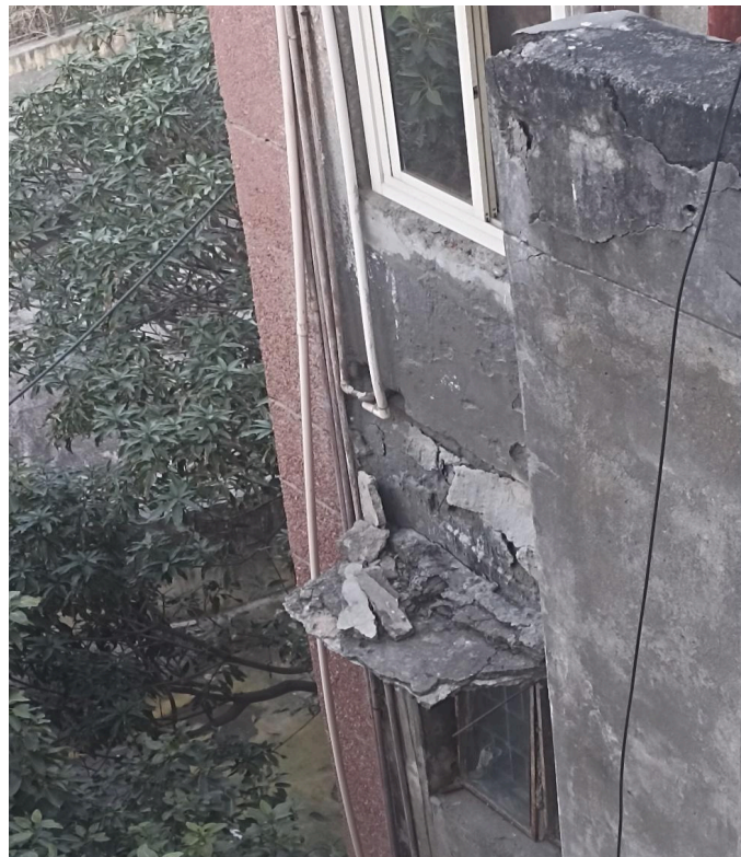
Image 12 : Showing severe damage at outer walls of building due leakage of water drainage system. (Image credits: Author)
