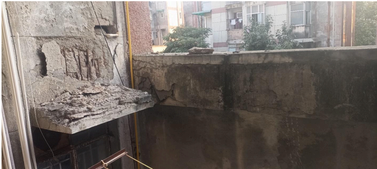
Image 9 : Showing severe damage to the connecting beam. (Image Credits: Author)
