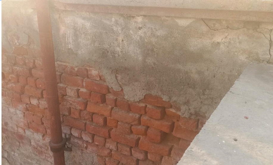
Image 8 : Showing Moderate decay of outer parapet walls due to rain water. (Image Credits: Author)
