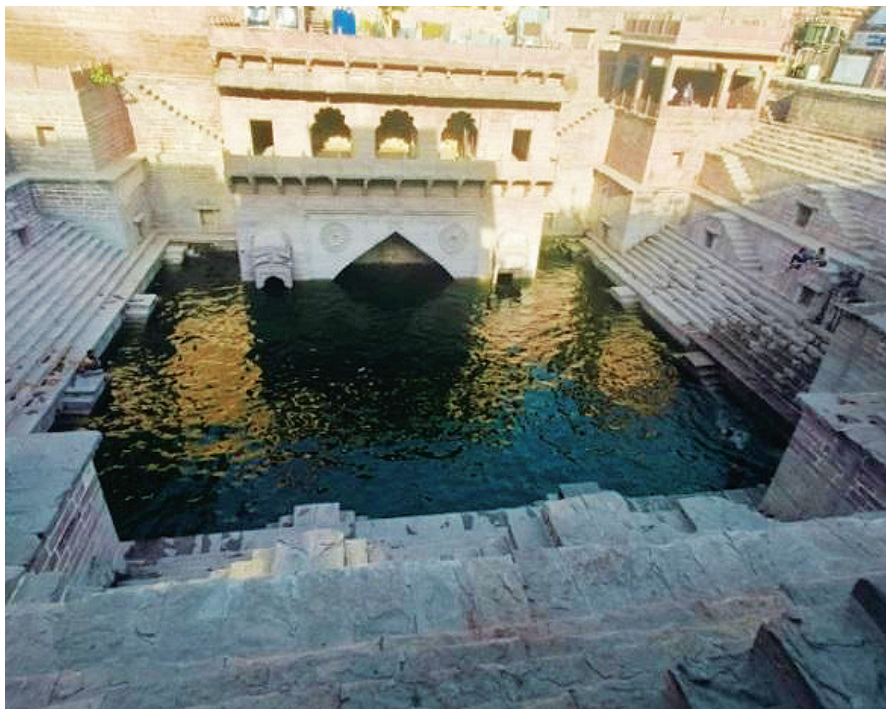
Fig. 18: Bawadi (Toorji ka Jhalra, Jodhpur in Rajasthan)
